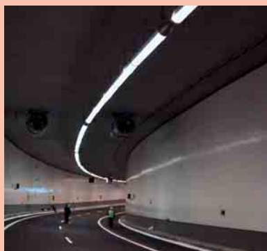
16 Light Pipe System
